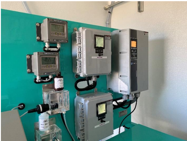
1 – RESIDUAL HQ CHLORINATION SKID CONTROL PANEL.
