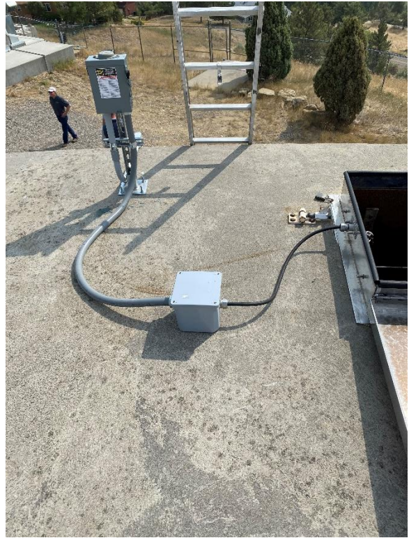
4 – ELECTRICAL CONNECTIONS AT NEW HILLTOP HATCH FOR MIXER
