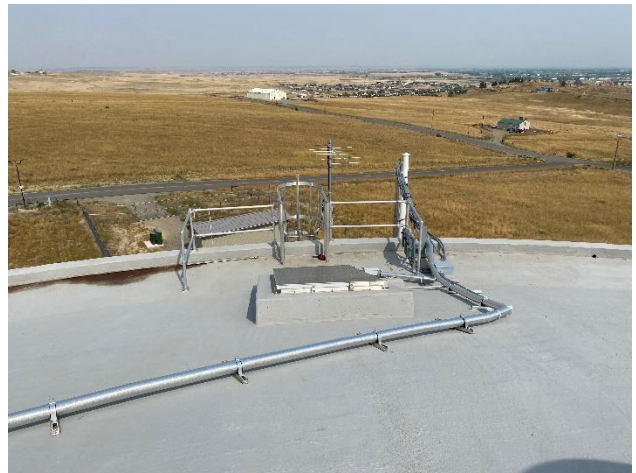
2 – PRIMARY HATCH AT OXBOW RESERVOIR.
